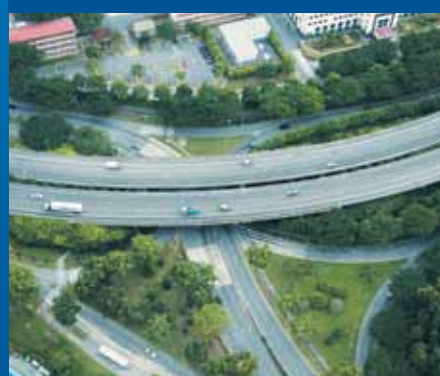
OKP's first design and build project at Bukit Timah Expressway.
