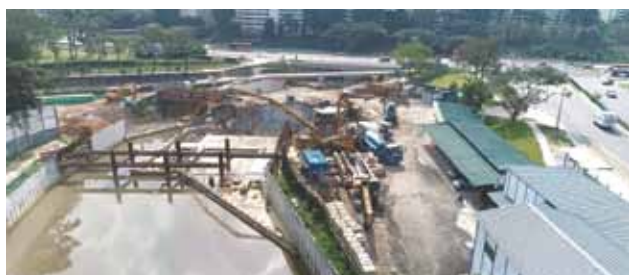
Chye Joo - Or Kim Peow JV is involved in the improvement to Bukit Timah first diversion canal from Holland Road to Clementi Road.
