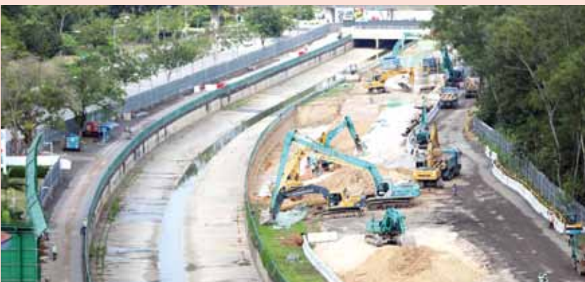
OKP is involved in improvement to Sungei Tampines (Tampines Ave 7 to Tampines Expressway).
