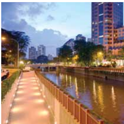
OKP completed the improvement to Alexandra Canal (between Zion Road and Kim Seng Road.)
