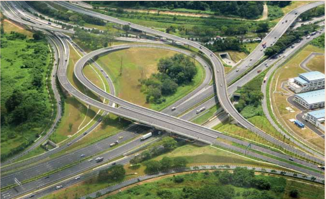
The expansion of the CTE/TPE/SLE interchange is one of OKP's completed projects.
