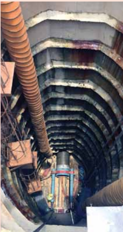
OKP is involved in constructing proposed sewers in Lim Chu Kang area – Contract 2.
