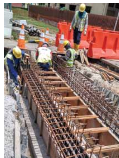
OKP won a contract for improvement to roadside drains V Contract E5 (Yishun Ave 1/6, Jalan Kembangan, Pasir Ris Estate and Hai Sing Estates areas).
