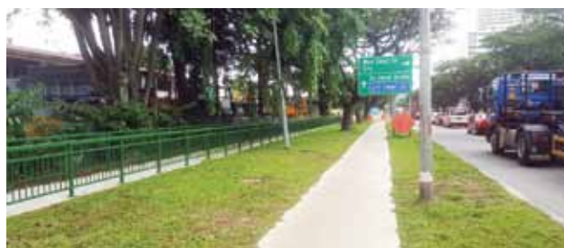
OKP completed the improvement to roadside drains V Contract 2 (Penjuru, Jalan Sampurna, Pioneer Sector and Jalan Buruh areas).
