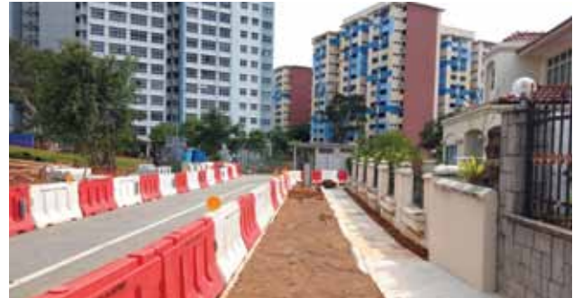
OKP is involved in improvement to roadside drains V Contract E5 (Yishun Avenue 1/6, Jalan Kembangan, Pasir Ris Estate and Hai Sing Estates areas).
