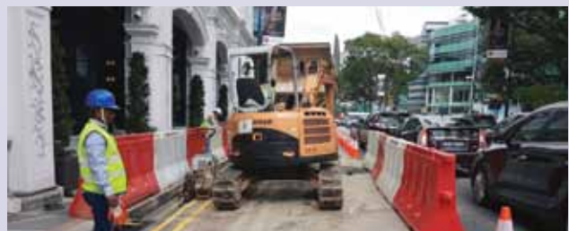
OKP won a contract for the improvement to roadside drains V Contract C5 (Stamford Road, River Valley Road, Upper Thomson Road and Burghley Drive).
