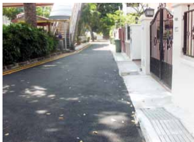
OKP completed the improvement to roadside drains V Contract C2 (Lorong 22 to 44 Geylang areas) in 2018.
