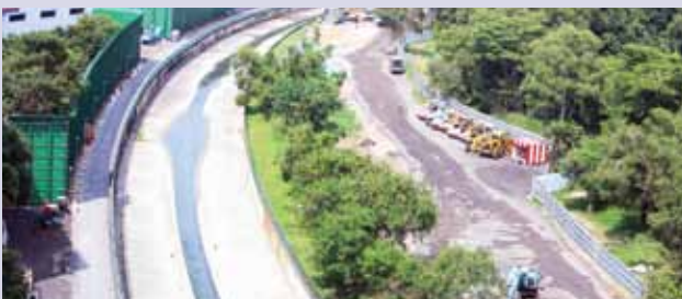
OKP is involved in the improvement to Sungei Tampines (Tampines Avenue 7 to Tampines Expressway).
