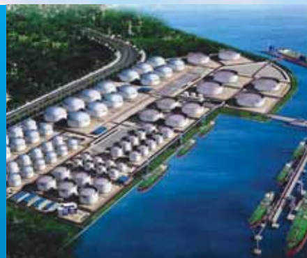
OKP completed its first and largest oil and gas-related project on Jurong Island.
