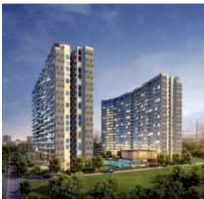
OKP co-developed LakeLife, a private condominium at Yuan Ching Road/Tao Ching Road in Singapore, which has been completed.
