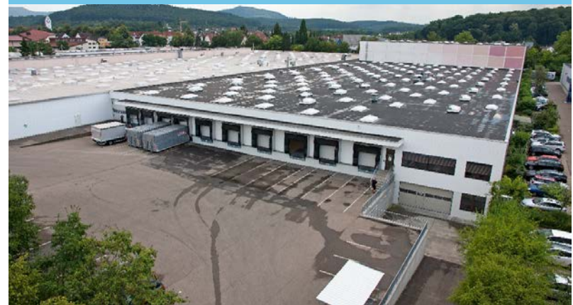
Logistikpark Stuttgart-Frickenhausen, Germany
