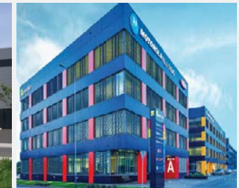
Green Office Kraków, Poland
