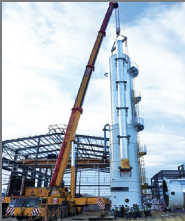
Location: Binh Son, Vietnam Scope of Work: Heavy Lifting Services Equipment: 500 Ton Mobile Crane
