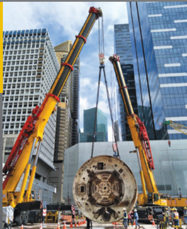
Location: Maxwell Road, Singapore Scope of Work: Heavy Lifting Services Equipment: 350/700 Ton Mobile Cranes
