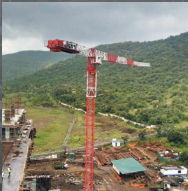
Location: Pune, India Scope of Work: Tower Crane Supply Equipment: 18 Ton Tower Crane
