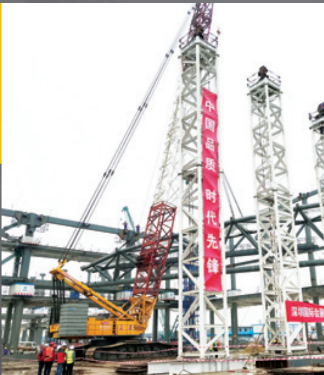
Location: Shenzhen, China Scope of Work: Heavy Lifting Services Equipment: 550 Ton Crawler Crane
