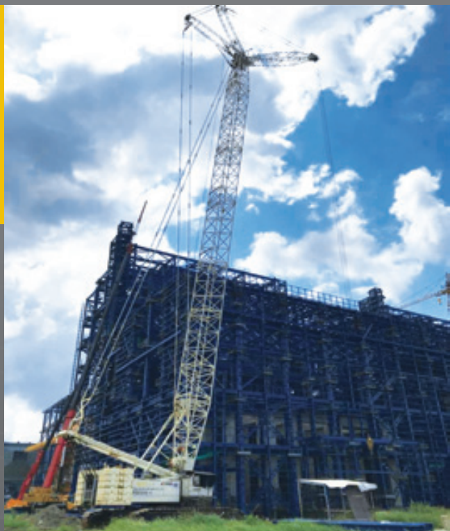
Location: Soc Trang, Vietnam Scope of Work: Heavy Lifting Services Equipment: 250 Ton Crawler Crane
