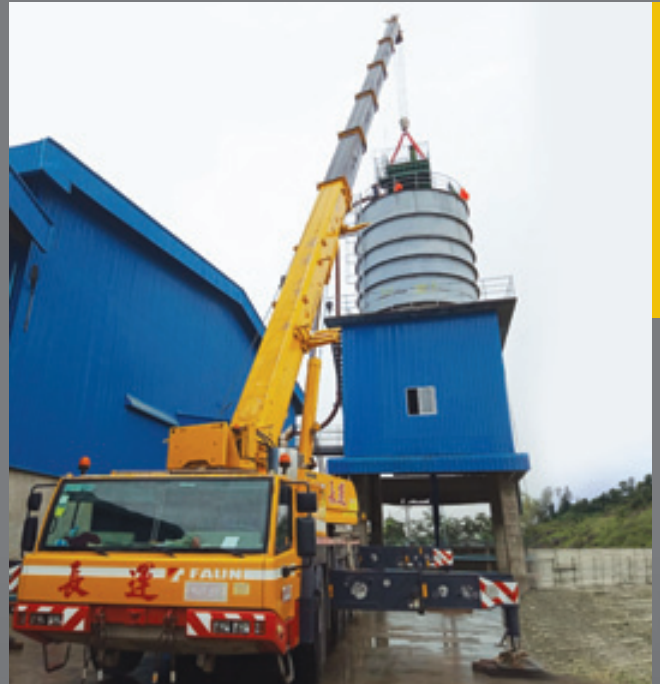
Location: Yangon, Myanmar Scope of Work: Heavy Lifting Services Equipment: 160 Ton Mobile Crane
