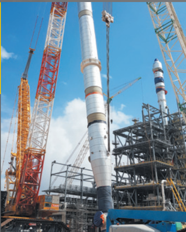
Location: Johor, Malaysia Scope of Work: Heavy Lifting Services Equipment: 1600 Ton Crawler Crane
