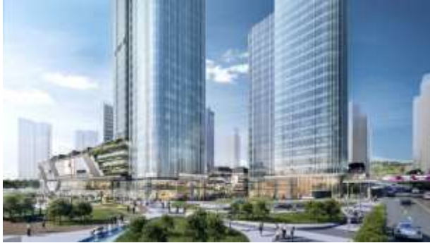
Yanlord Reverie Plaza, Shenzhen, 仁恒梦创广场, 深圳 Office & Retail Total GFA: 209,440 sqm (in which 60,000 sqm held under investment property)
