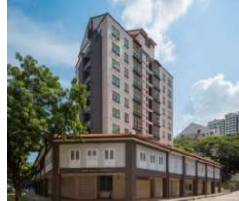
Park Avenue Robertson Service Apartment: 36 rooms GFA: 3,286 sqm (35,374 sqf)
