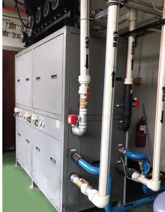
Heat recovery system installed at one of the Group's factories in Malaysia.
