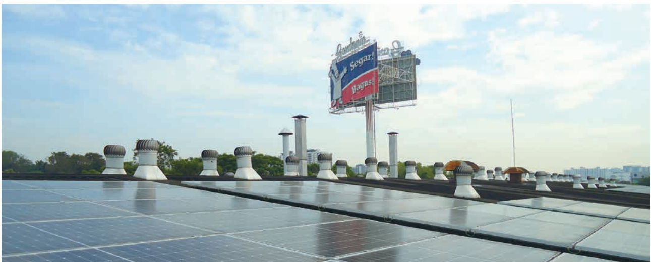
Solar panels installed on the rooftop of one of the factories of our joint venture in Malaysia.
