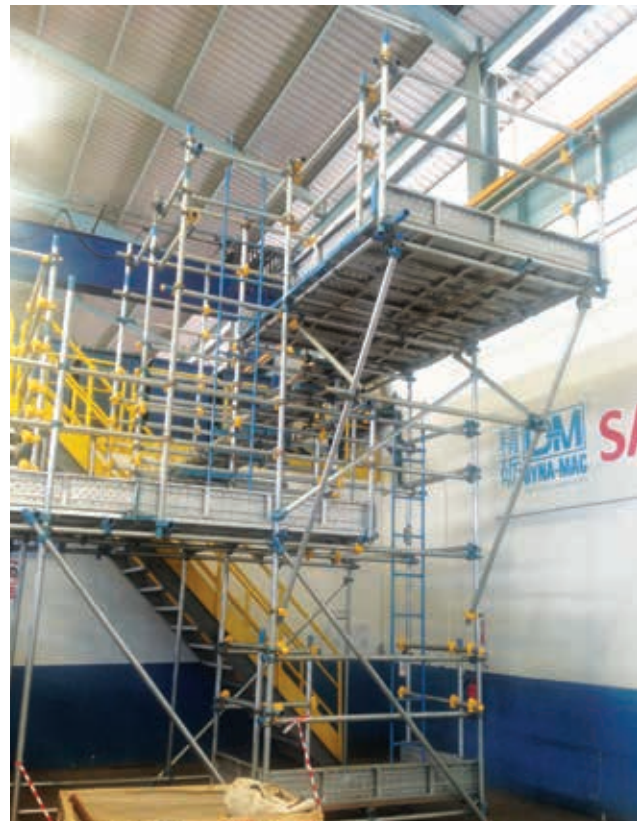
In-house mock-up scaffold platform
