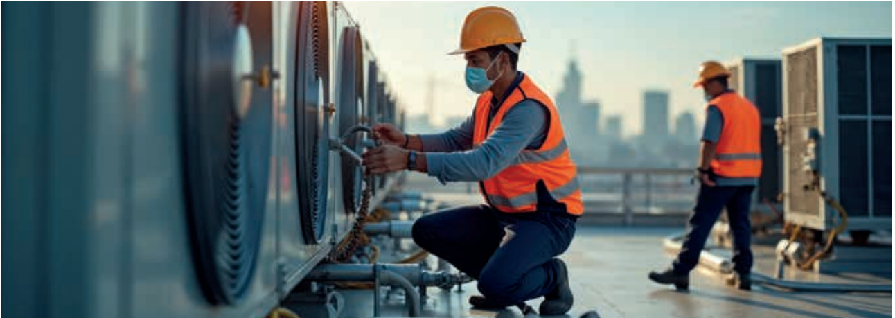
Commercial Aircon servicing in progress
