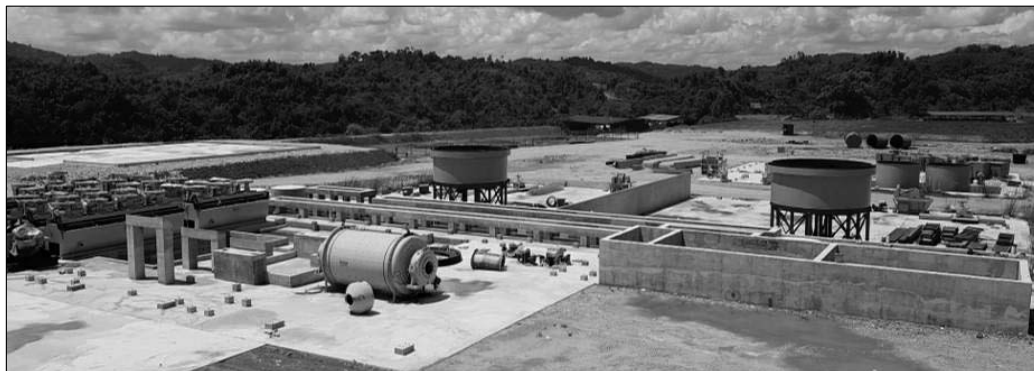
Figure 3.3 Construction of Sokor flotation plant – October 2019
