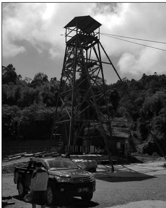
Figure 3.4 Ketubong shaft headframe – October 2019
