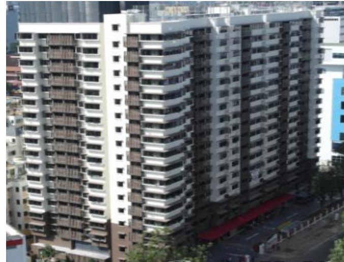
New dormitory block at Westlite Toh Guan
