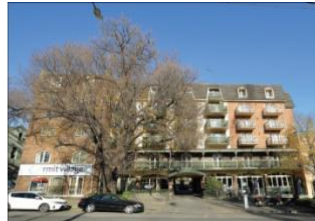
External Façade of RMIT Village
