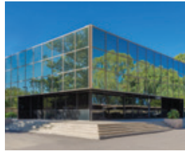
3 2601 West Broadway Road, Tempe
