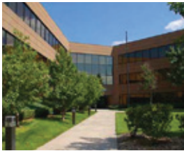
11 11900 East Cornell Avenue, Denver
