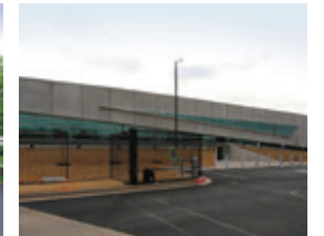
35 4121 & 4114 Perimeter Center Place, Oklahoma City
