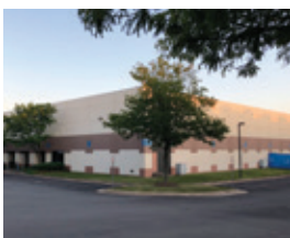
56 45901-45845 Nokes Boulevard, Northern Virginia
