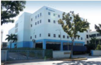
98 2A Changi North Street 2
