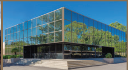
2601 West Broadway Road, Tempe
