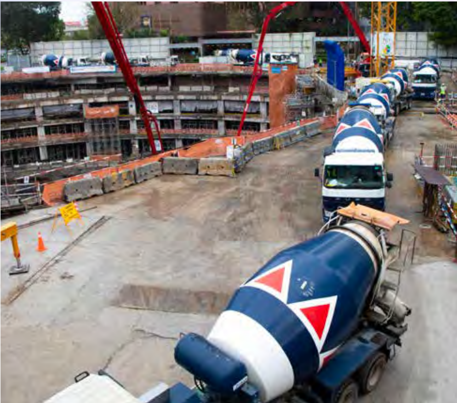
The AiR Digital system effectively managed the complex logistics of The Skywaters raft foundation mass pour including fleet optimisation, auto-replenishment of raw materials and truck queueing (see page 13).
