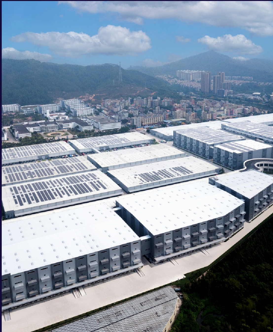
Goodman Huiyang Industrial Park, Huiyang, China
