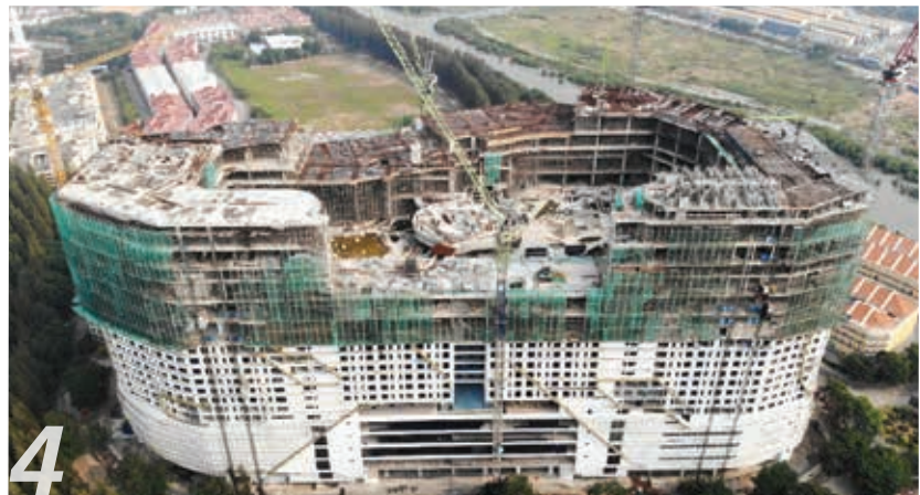
1 - Water Theme Park 2 - Retail Floor 3 - Overview Building (Day View) 4 - Construction Progress as at September 2019
