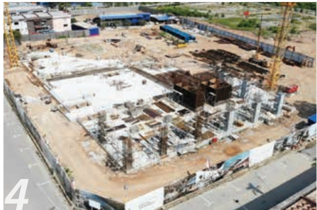
1 - Overview Building (Day View) 2 - Swimming Pool 3 - Spa 4 - Construction Progress as at September 2019
