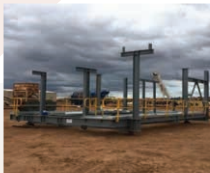
Structural Steel Assembly
