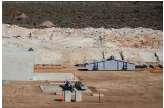
Feed Bin Walls and Equipment Pads
