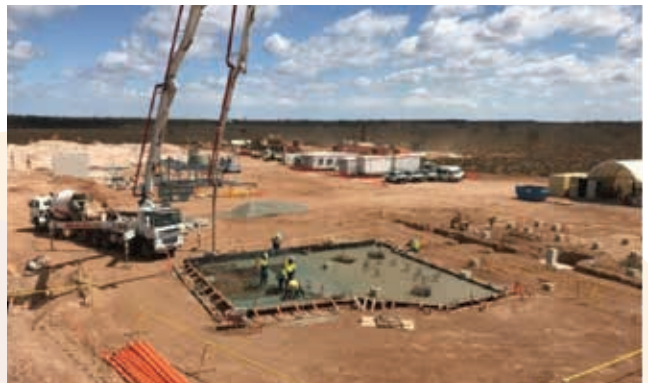
DMS Plant Slab
