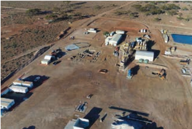
Bald Hill project construction aerial view
