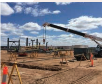
Structural Steel Assembly
