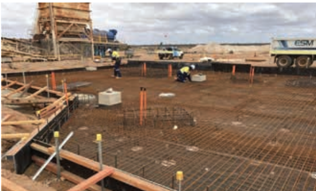
DMS Plant Slab
