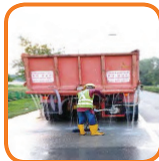
Road washing using recycled water
