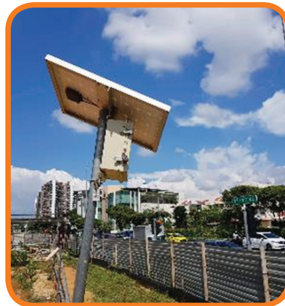
Solar source for our noise monitoring system
