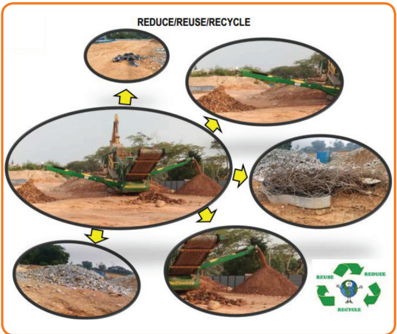
Separation of Soils/Rock/Stones/Rebar for reuse by our High Efficiency Screener
