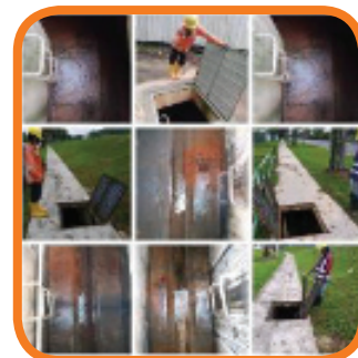
Recycled water for Drainage washing
