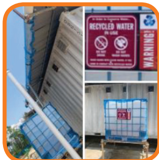
Collection of rain water into IBG Bin for cycling purposes
