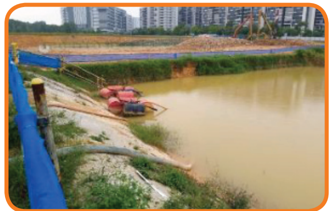
Use of sustainable material LSS for slope protection
