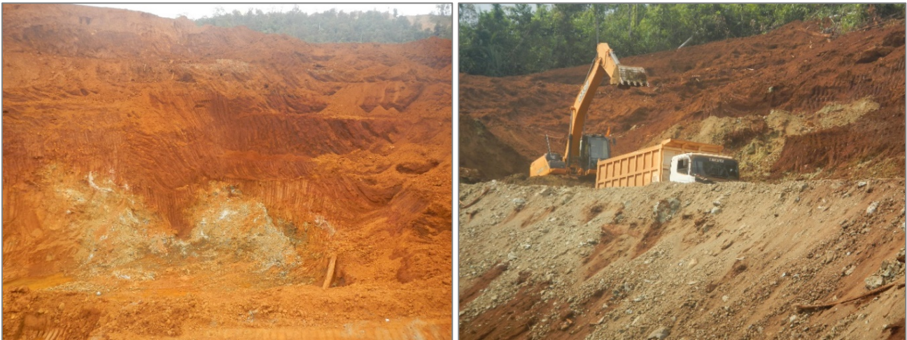
Figure 11-1. Example of mining operations, September 2018.
