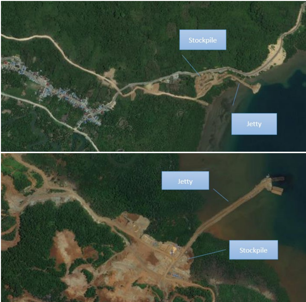
Figure 12-1. Jetty and stockpile infrastructure at Torete (top) and Buleleng (bottom).
