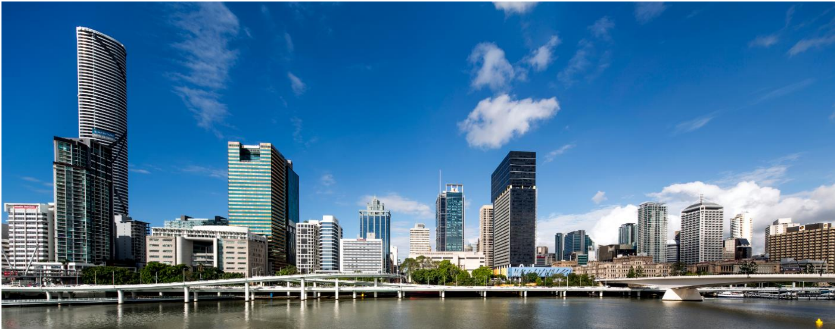
275 George Street in Brisbane saw improved committed occupancy
