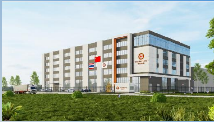
Mansfield (Thailand) Co., Ltd. Rayong, Thailand Built-in area: 20,800 sqm
