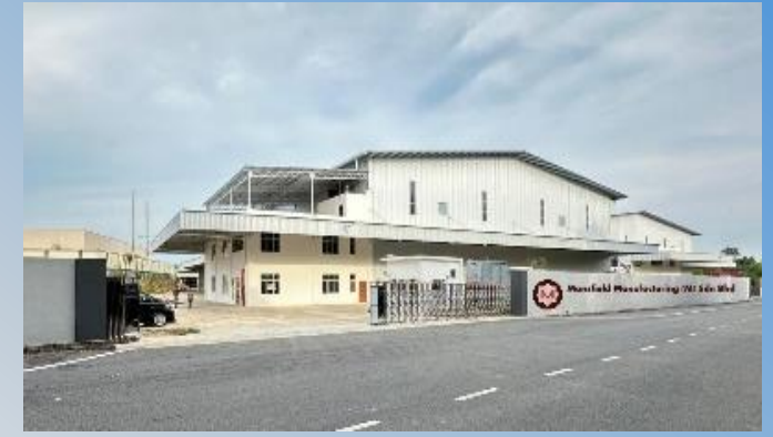
Mansfield Manufacturing (M) S/B Melaka Built-in area: 10,000 sqm
