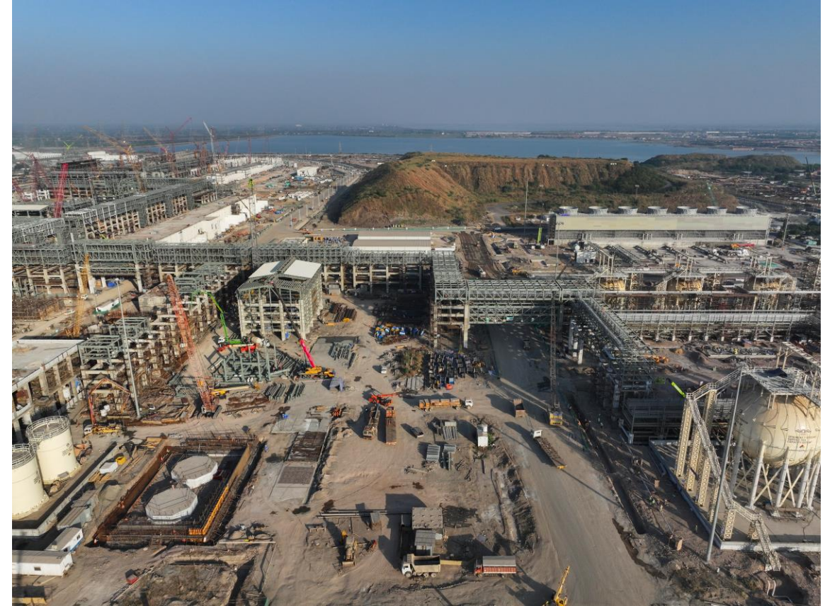
Construction in Progress
