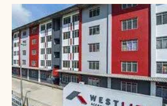
Westlite Senai, Johor Malaysia – assessment in progress
