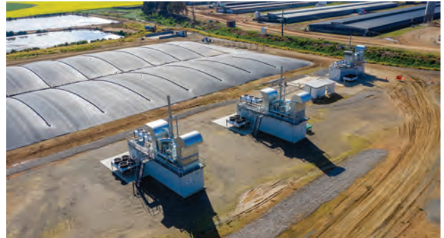
Rivalea's biogas power generators at Corowa, New South Wales.
