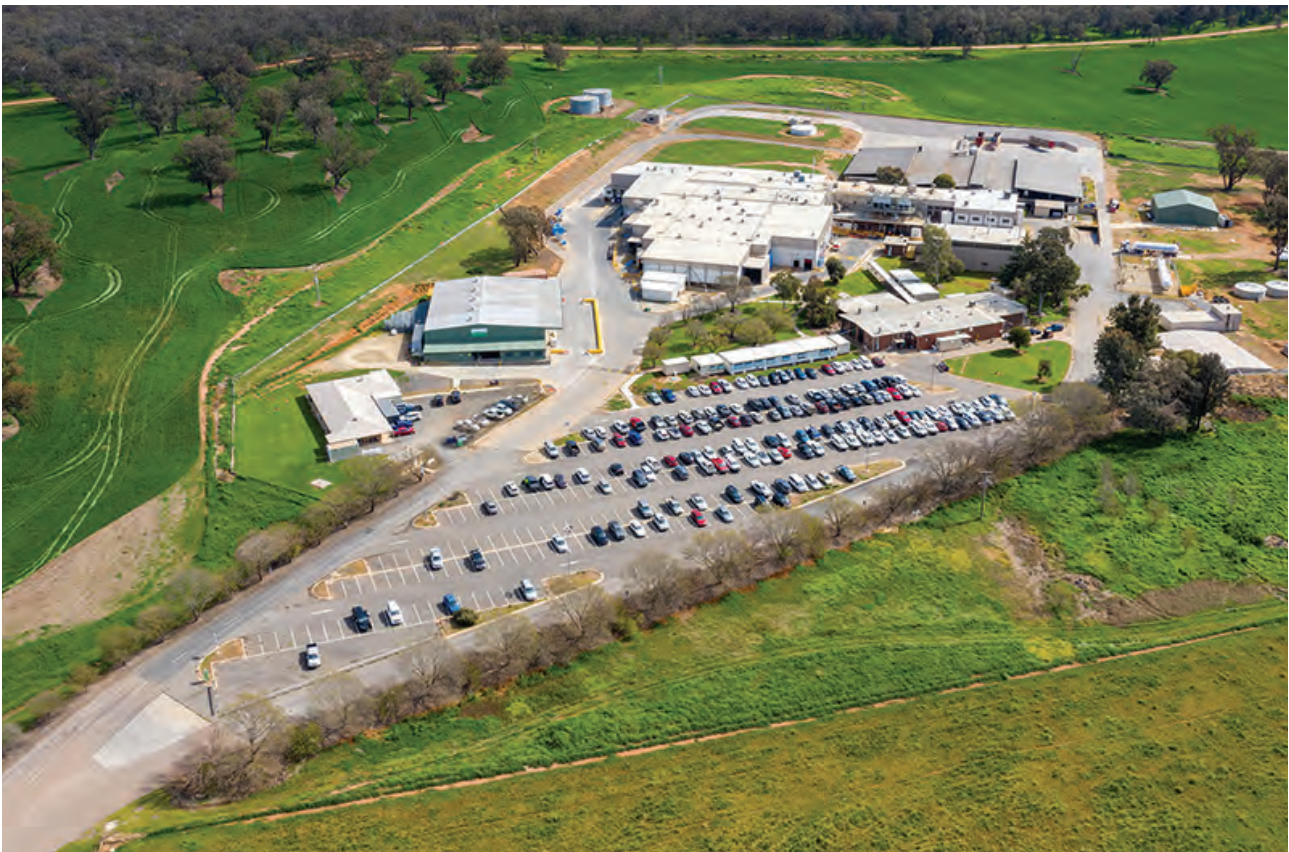
Rivalea’s meat processing facility at Corowa, New South Wales.
