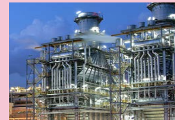
A top-tier gas-fired power plant in Singapore
