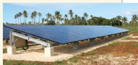
A solar power generation facility in Tonga
