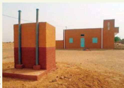
An improved ventilated toilet. The toilet, neatly painted to match the color of the nearby house, is properly maintained by local residents.
