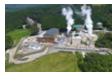
Otake Power Station
