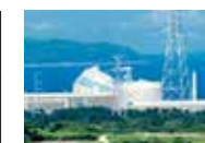
Genkai Nuclear Power Station
