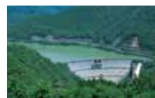
Hitotsuse Power Station
