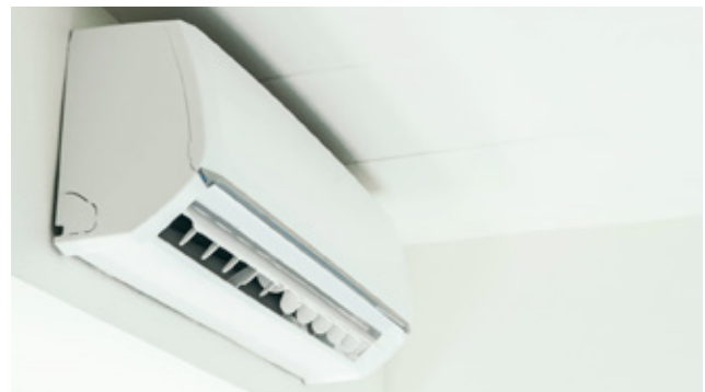
Sensor monitoring of lighting and air-conditioning
