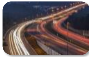
Transurban Queensland Toll Road
