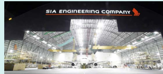
After Replacement – Average 750lux. The lighting system is dimmable and the lighting levels are preset to 500lux and 750lux.
