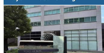
Toyo MK Fuso Building
