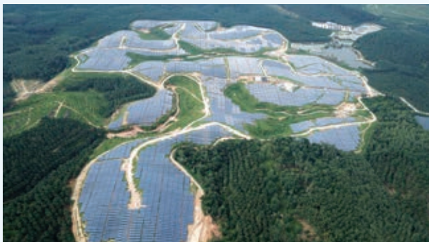
Sinar Kamiri is committed to support the development of clean energy.
