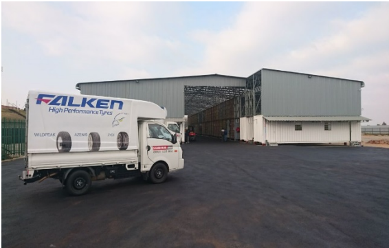
New container warehouse in Johannesburg, South Africa
