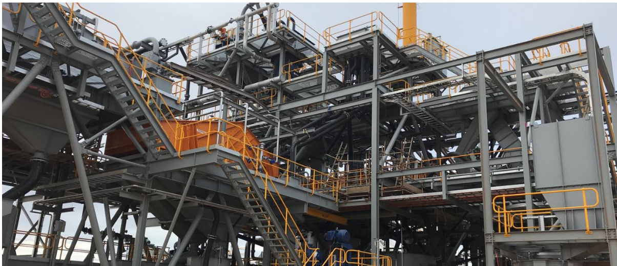
Above: picture of recently commissioned Bald Hill processing plant, built by Primero
