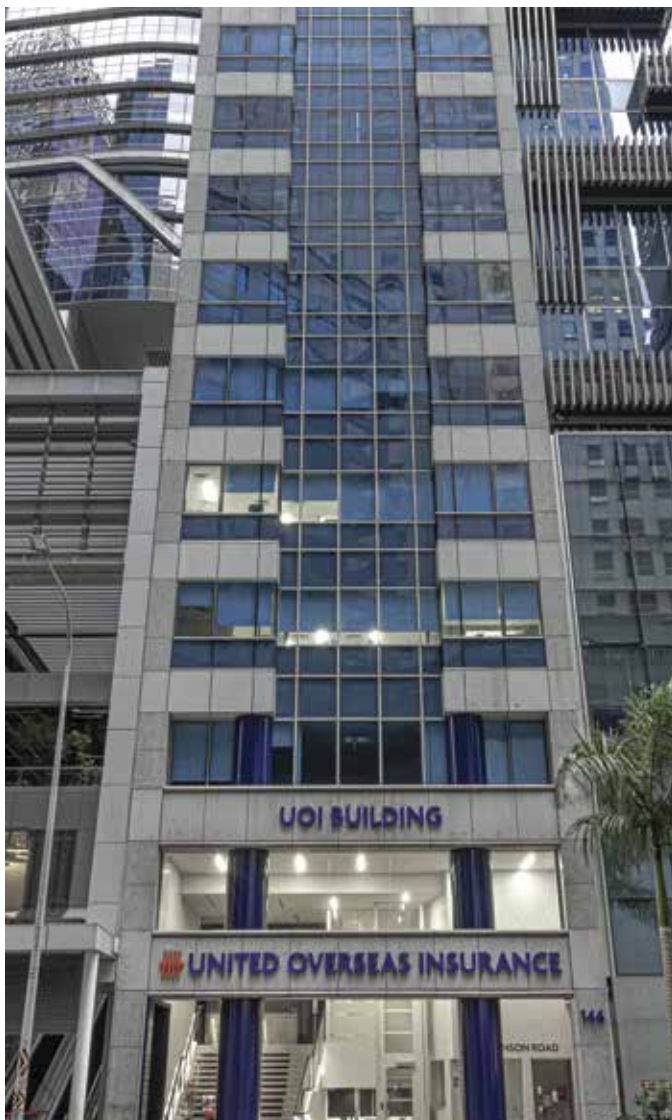
A prominent street front along Robinson Road.
