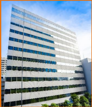
Omori Prime Building (Tokyo)
