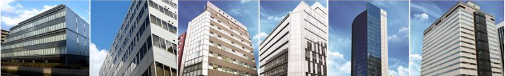
(Left to right) IXINAL Monzen-nakacho Building (Tokyo), Higashi-nihonbashi 1-chome Building(Tokyo), TS Ikebukuro Building(Tokyo), ABAS Shin-Yokohama Building (Yokohama), SII Makuhari Building (Chiba), Fujitsu Makuhari Building (Chiba) (collectively known as "Existing Japan Properties")
