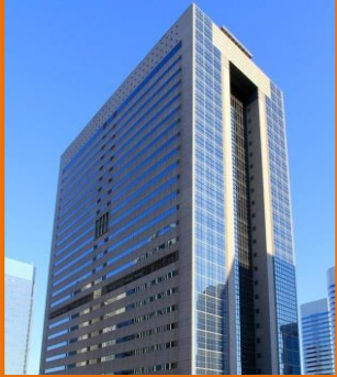
mBay Point Makuhai Building (Chiba)
