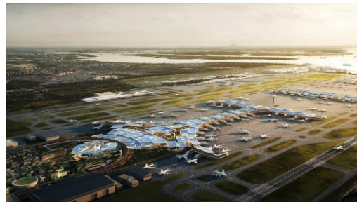
Construction of Changi Airport Terminal 5 to commence in 2025
