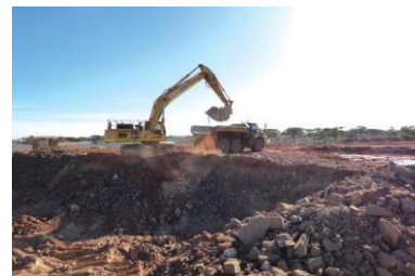
Expansion of Tailing Storage Facility
