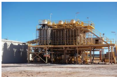
Spirals installed in Process Plant (Feb 2015)
