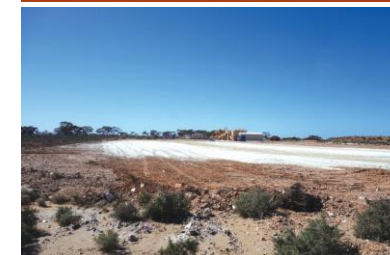
The completed ROM pad
