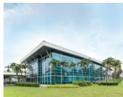
3 Tuas South Ave 4
