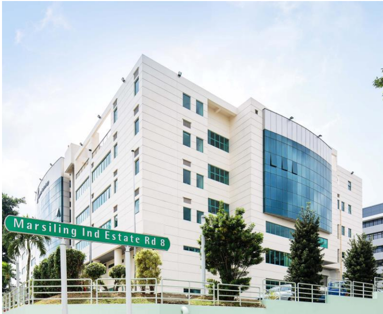
30 Marsiling Industrial Estate Road 8
