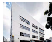
60 Tuas South Street 1
