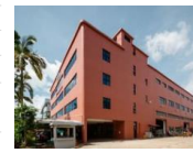
31 Changi South Ave 2
