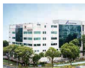
30 Marsiling Industrial Estate Road 8
