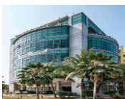
2 Tuas South Ave 2
