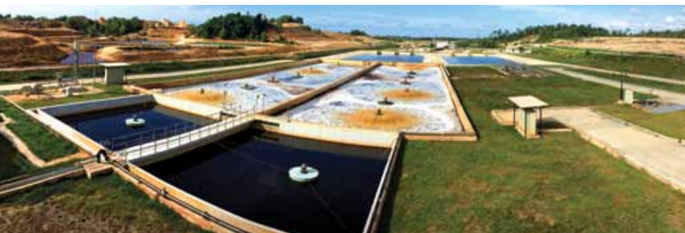
An Integrated Waste Management System was successfully delivered to the Brunei Economic Development Board in March 2016.
