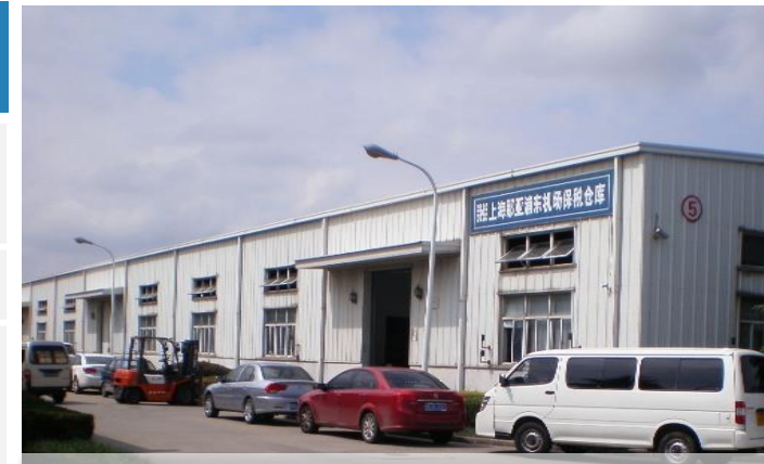
Ouluo Logistics Centre before redevelopment
