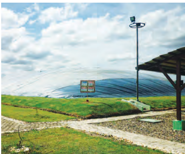
Reducing GHG emissions: a methane capture facility and biogas engine to generate electricity
