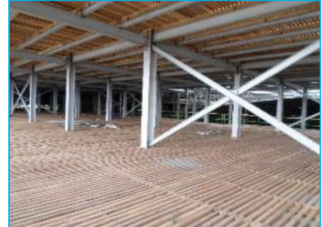
New hanging shed
