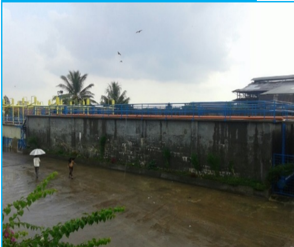
Waste water treatment plant
