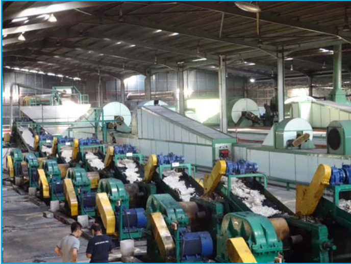
SMR line renovation
