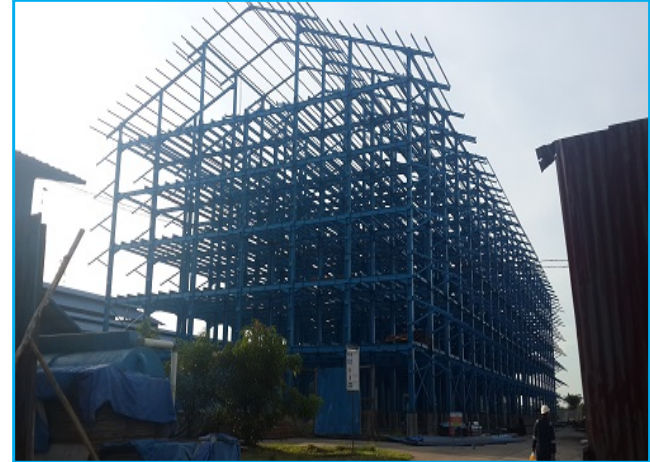
Hanging shed B
