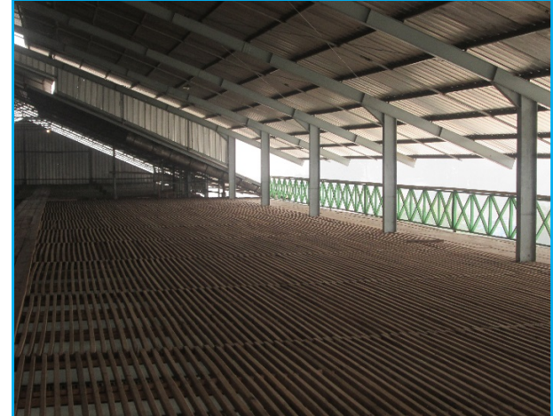
Hanging shed extension
