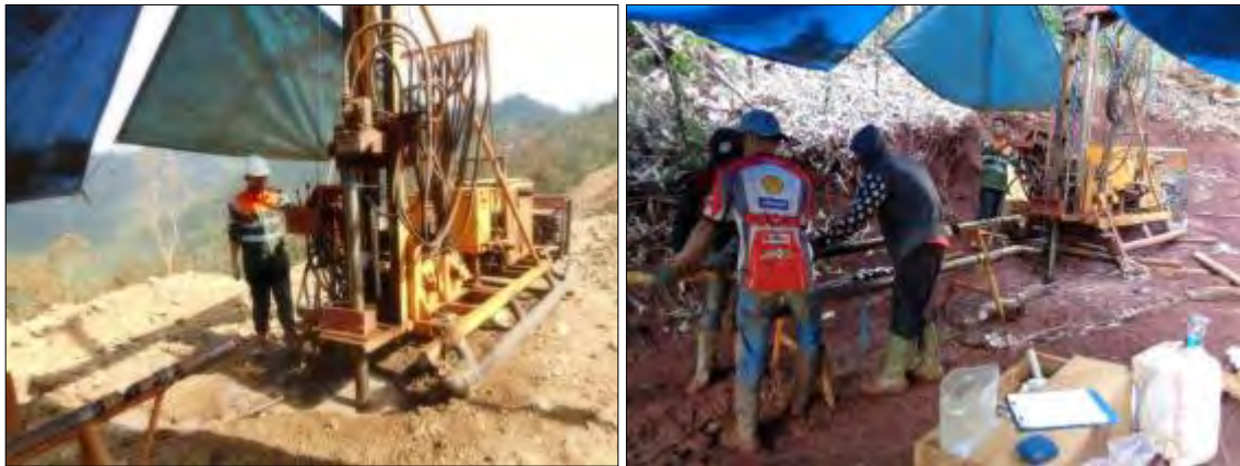
Figure 6.1 Drilling Activities using Jacro-175 with Triple Tube Core-barrel
