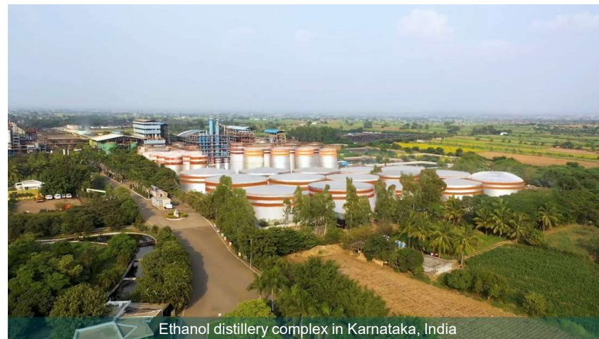
Ethanol distillery complex in Karnataka, India
