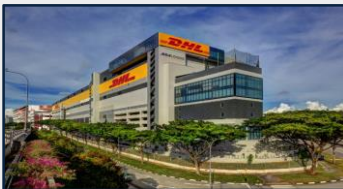
10 DHL Supply Chain ARC 1 Greenwich Drive
