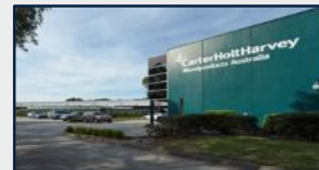
24 41 – 45 Hydrive Close, Dandenong South
