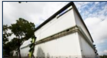
2 ALOG Cold Centre 2 Fishery Port Road
