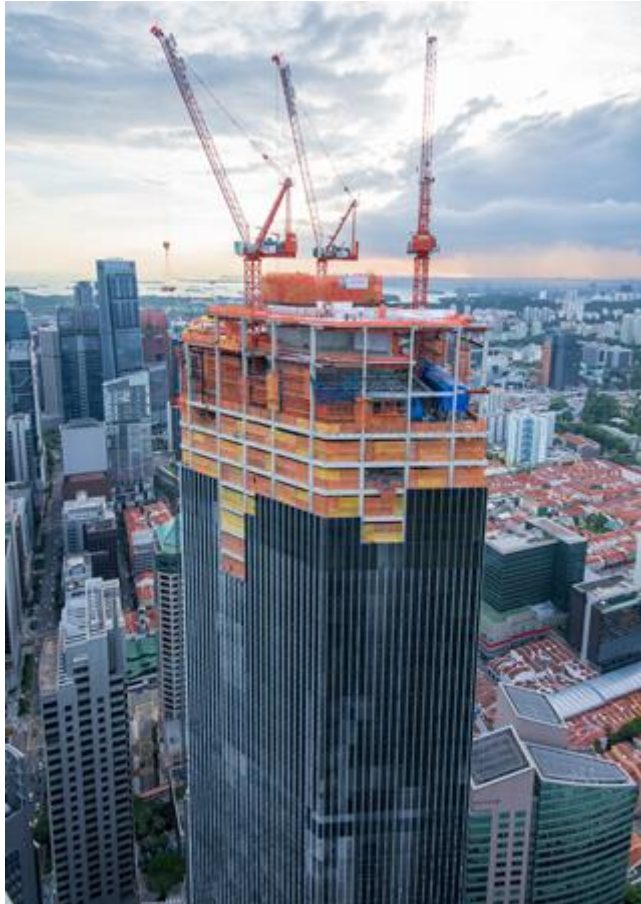
CapitaSpring topping-out at level 51
