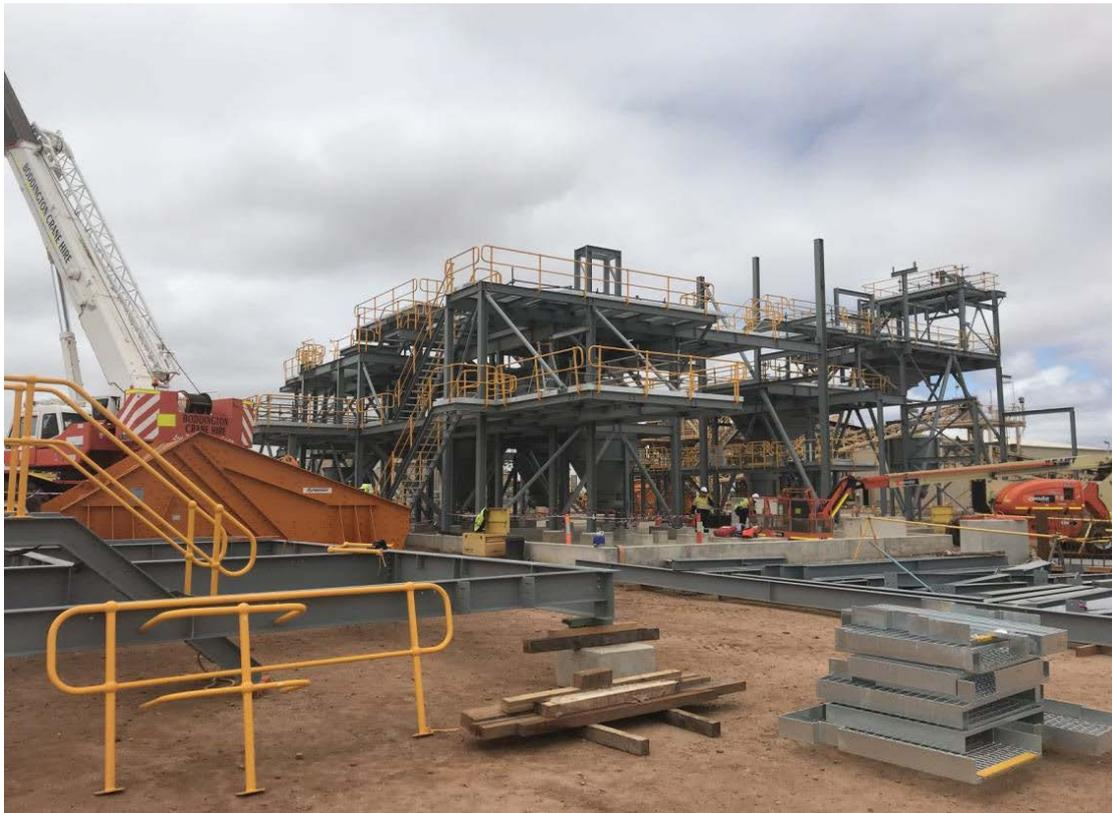
Figure 2 - Underflow hoppers and screen decks being installed
