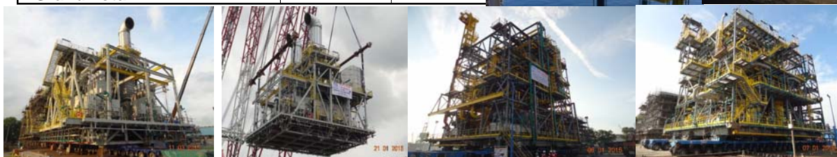
Ten Tullow TS Power Generation
