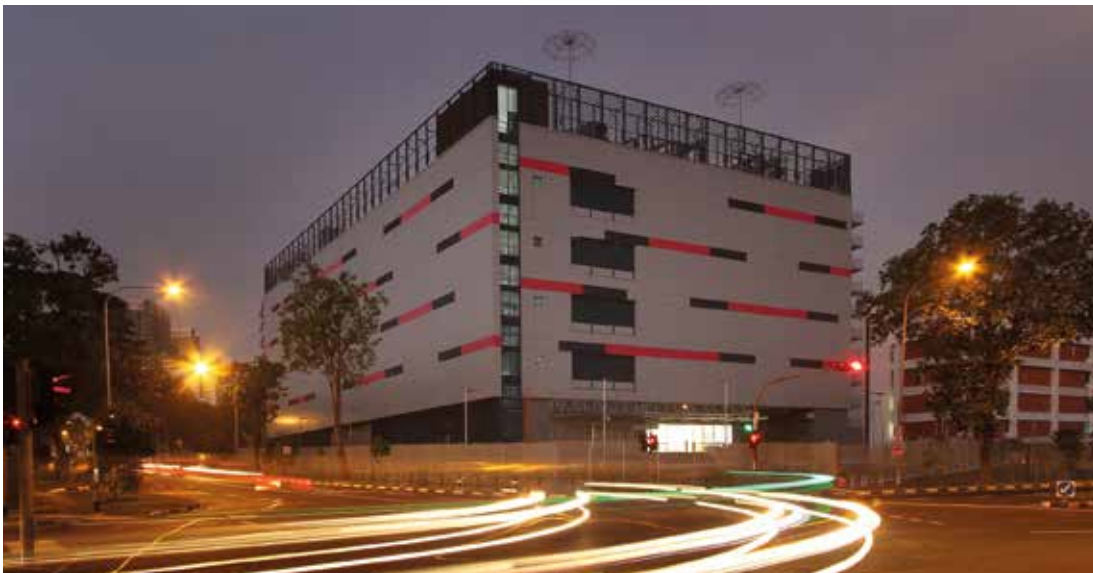
DC1 is a purpose-built five-storey data centre facility located outside the Woodlands Regional Centre.
