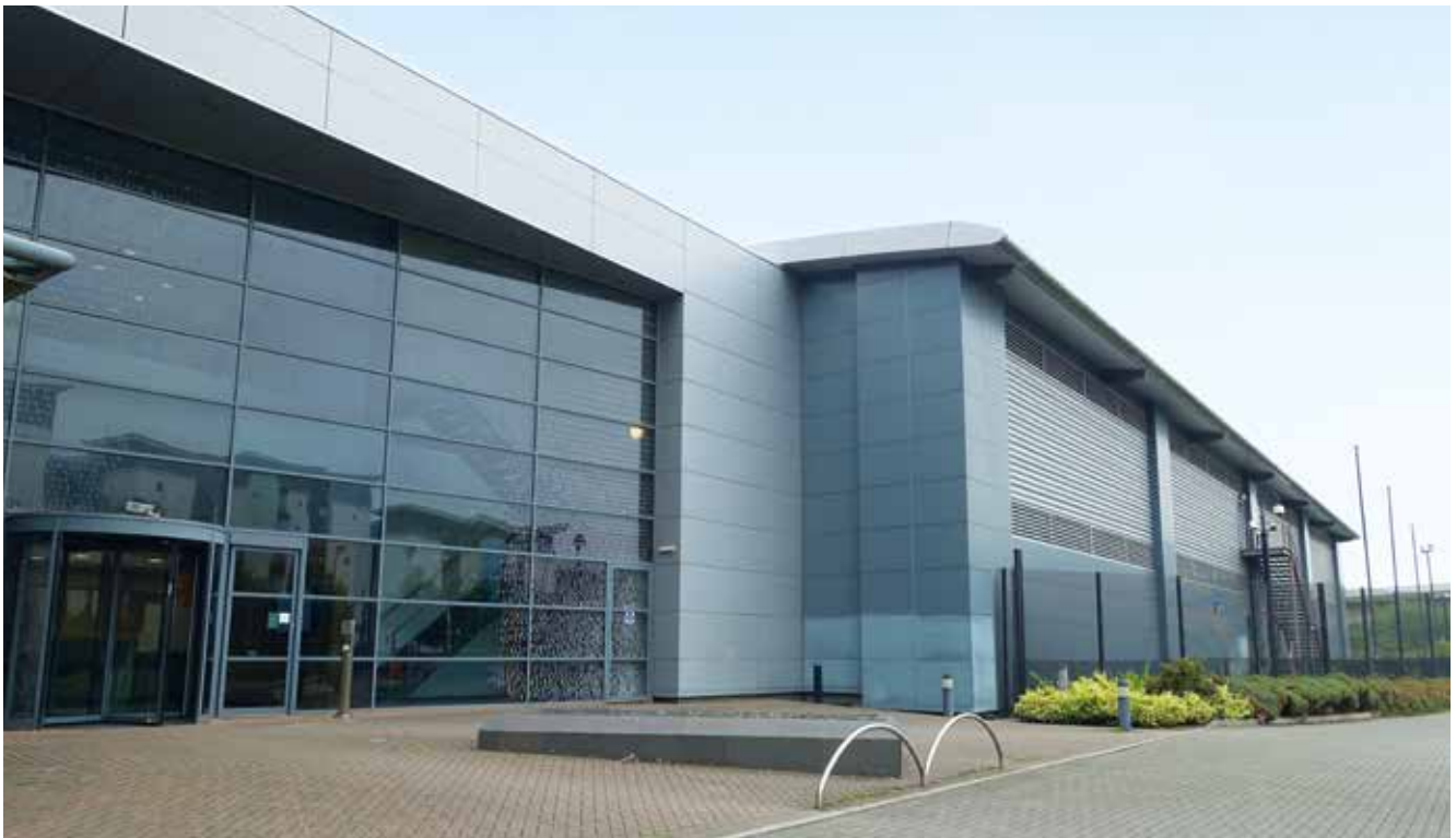
Cardiff Data Centre is strategically situated within the Celtic Gateway Business Park.
