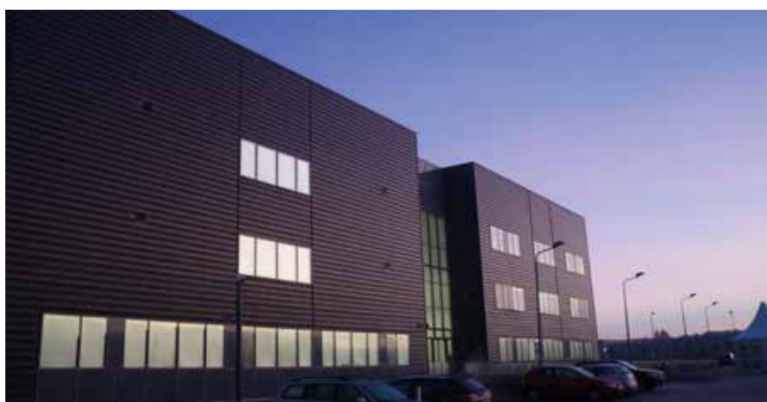
With connection to North America and Europe via submarine cables, Almere Data Centre provides a highly-connected and secure environment for clients.
