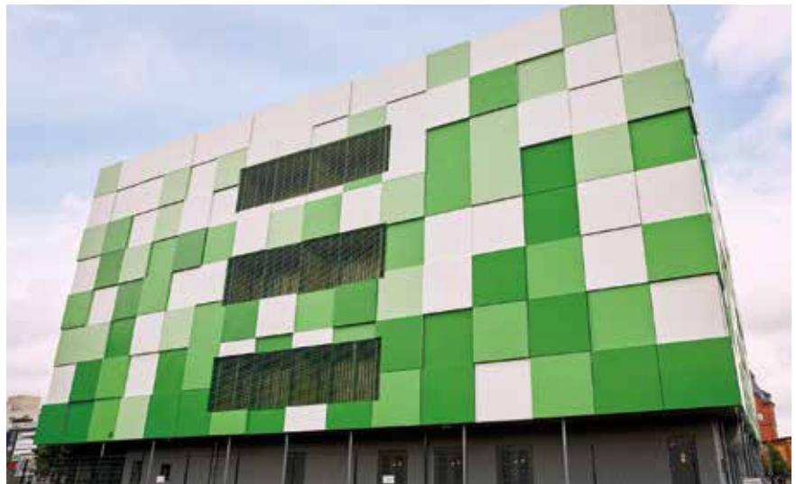
maincubes DC is located within a data centre hub and offers high interconnectivity to the world's leading internet exchange point, DE-CIX.
