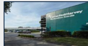
24 41 – 45 Hydrive Close, Dandenong South
