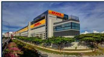
10 DHL Supply Chain ARC 1 Greenwich Drive
