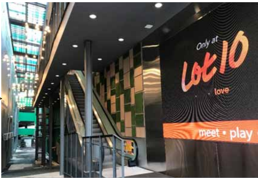
The new escalator improves accessibility to the mall from the new MRT station exit
