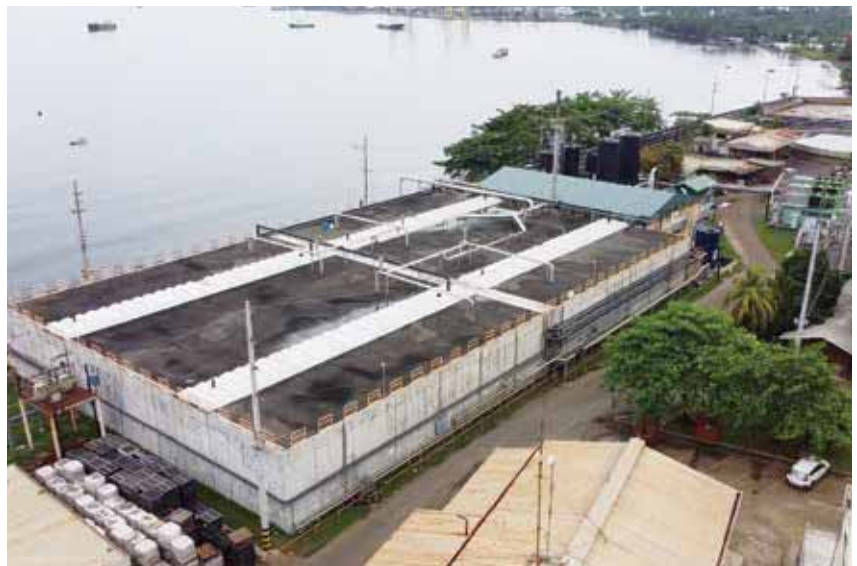
The cannery’s waste-to-energy facility in Bugo, Cagayan de Oro City
